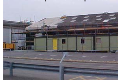
UKAEA roof prior to encapsulation
